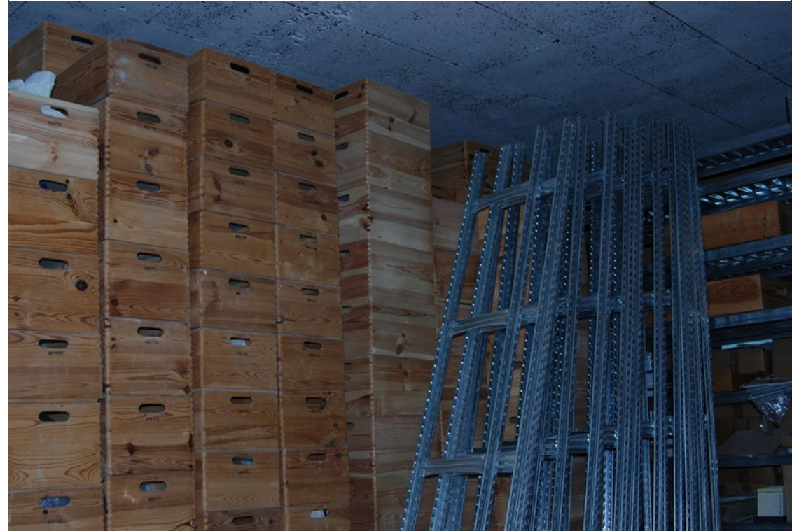
The Practicothèque under construction, Brussels, 2022. Photography courtesy of Lotte Bode
